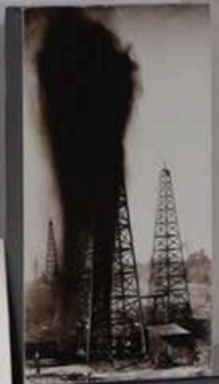
Oil Wells c. 1920s Louisiana Department of Conservation Homer Field Blossom sand well flowing 30,000 barrels a day State Library of Louisiana
